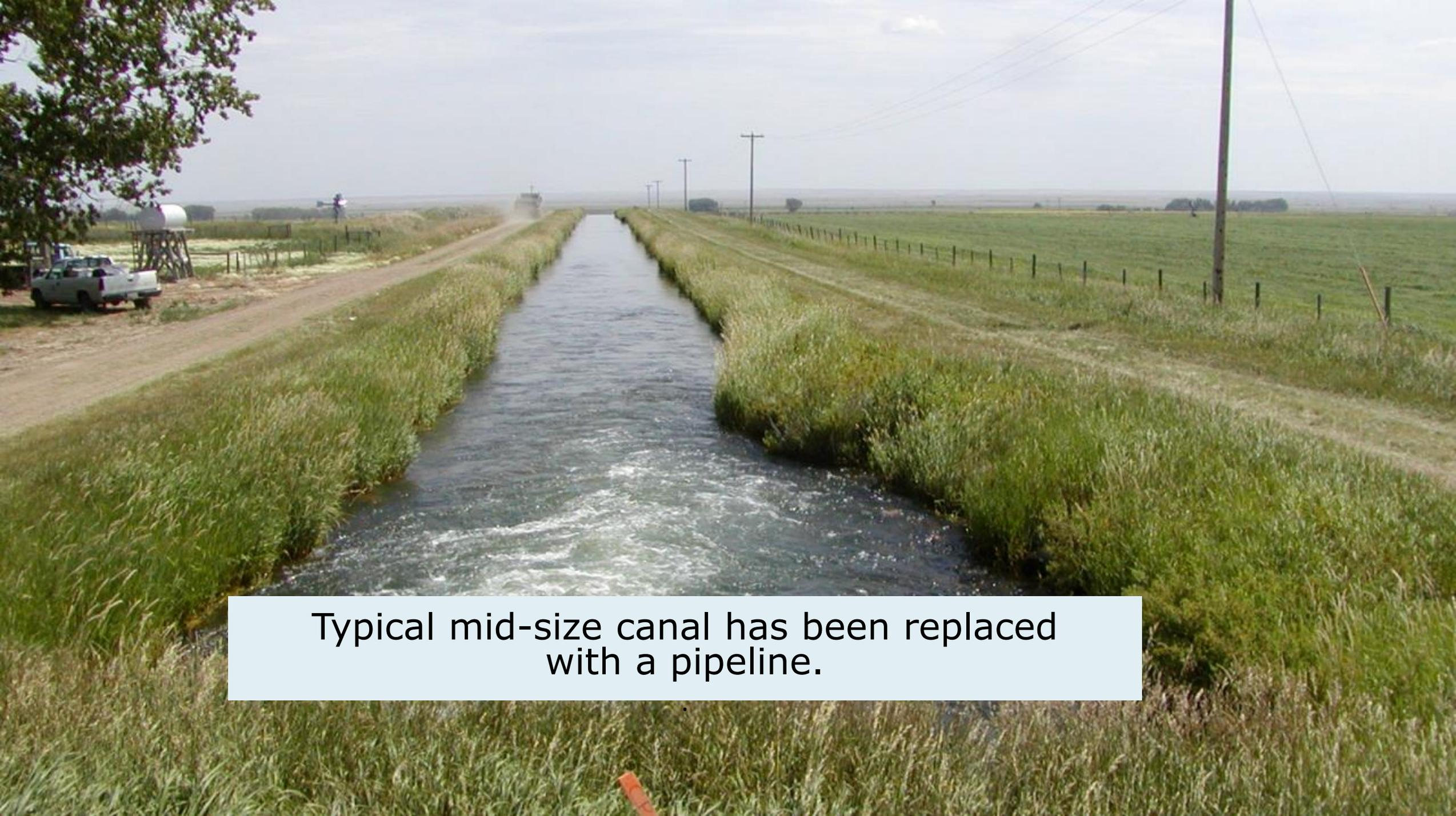
Typical mid-size canal has been replaced with a pipeline.
